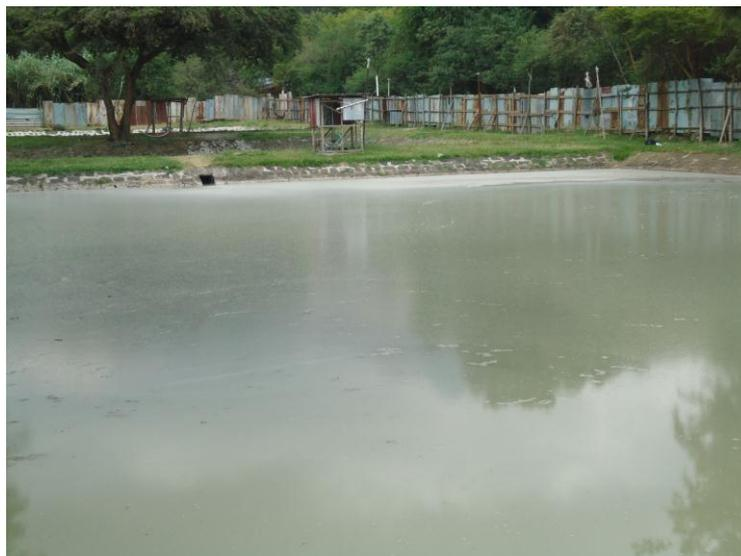
**Figure 2.** Partial view of facultative pond at Meta Abo Brewery wastewater treatment system
